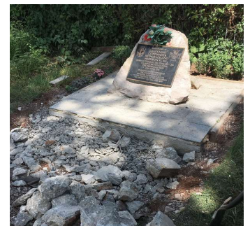
Refurbishment under way
