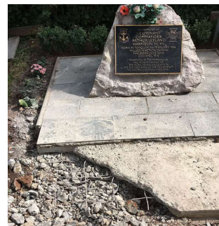
Before & During Refurbishment
