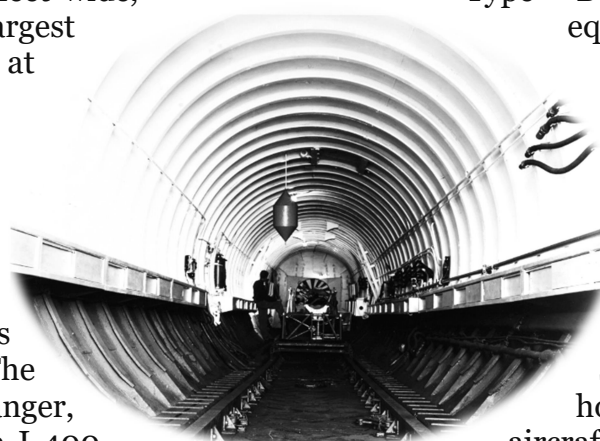
Inside of the hangar in sail
