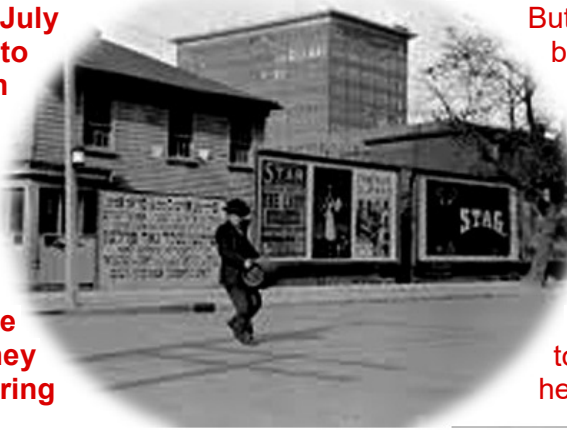
A man carrying keg during prohibition September 1916
